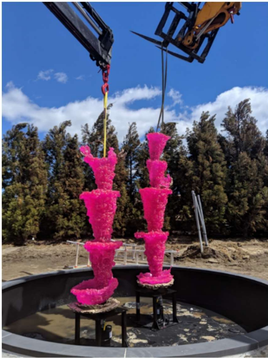
Lynda Benglis Rigging & Installation
